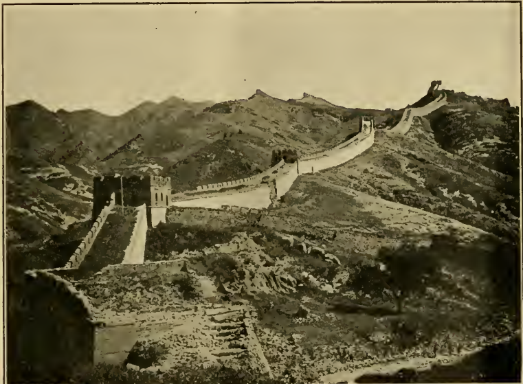
THE OLD AND THE NEW. TELEGRAPH LINE ON THE GREAT WALL OF CHINA.
